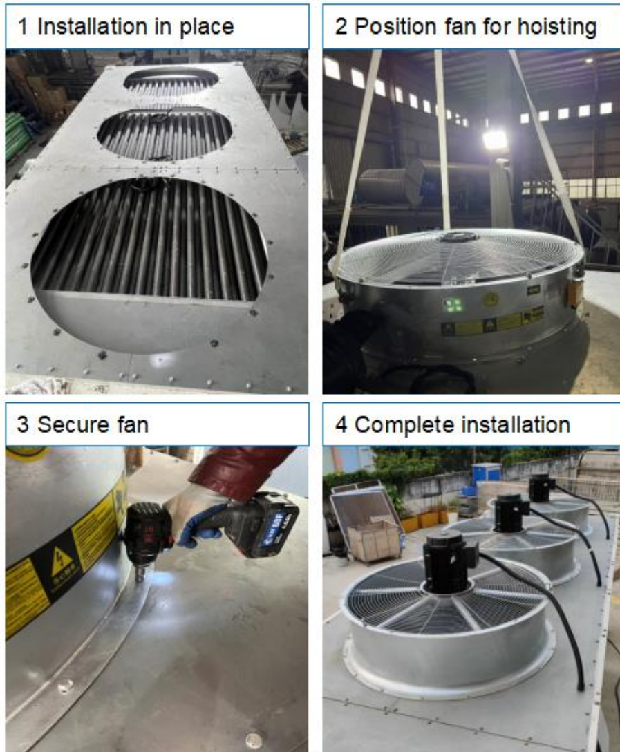
Figure 7-8 Schematic for Fan Installation
