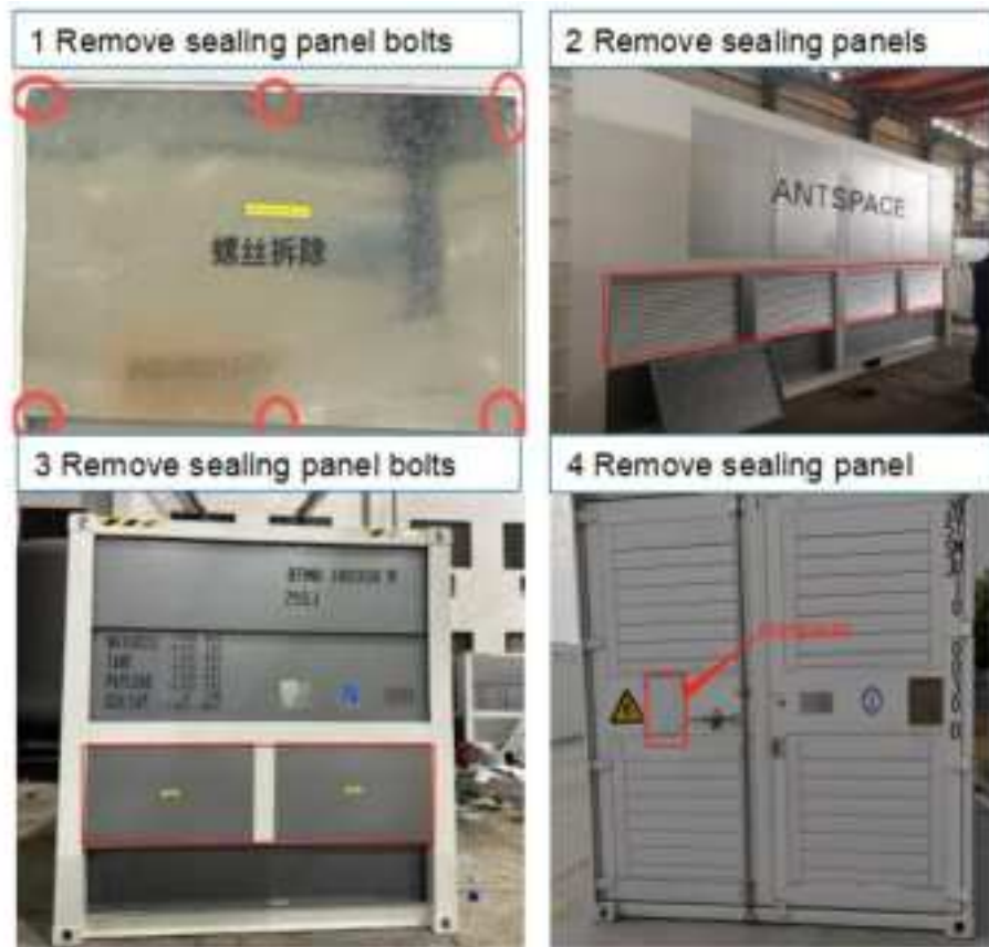
Figure 7-4 Schematic for Removing Side Sealing Panels
