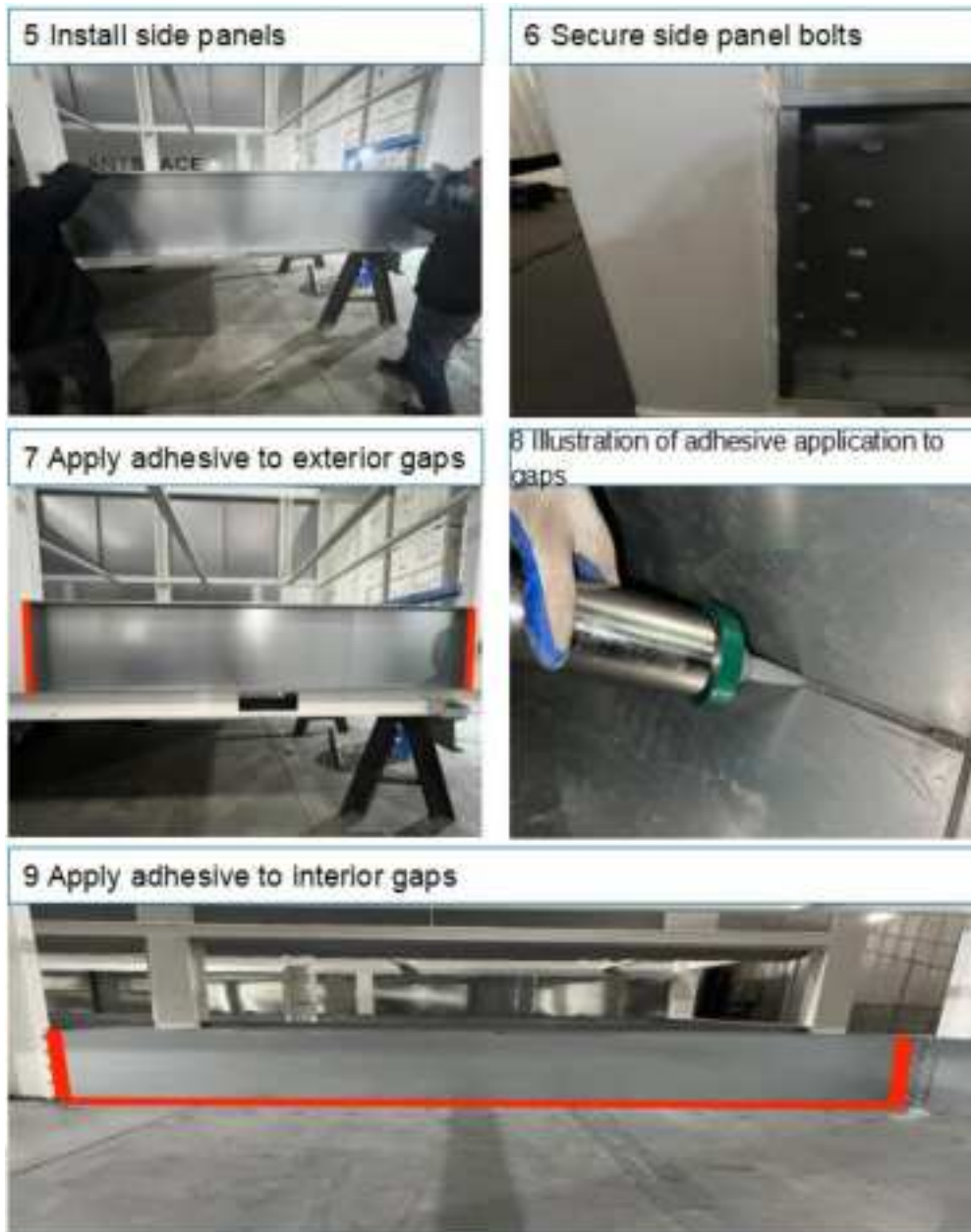
Figure 7-7 Schematic for Side Panel Installation
