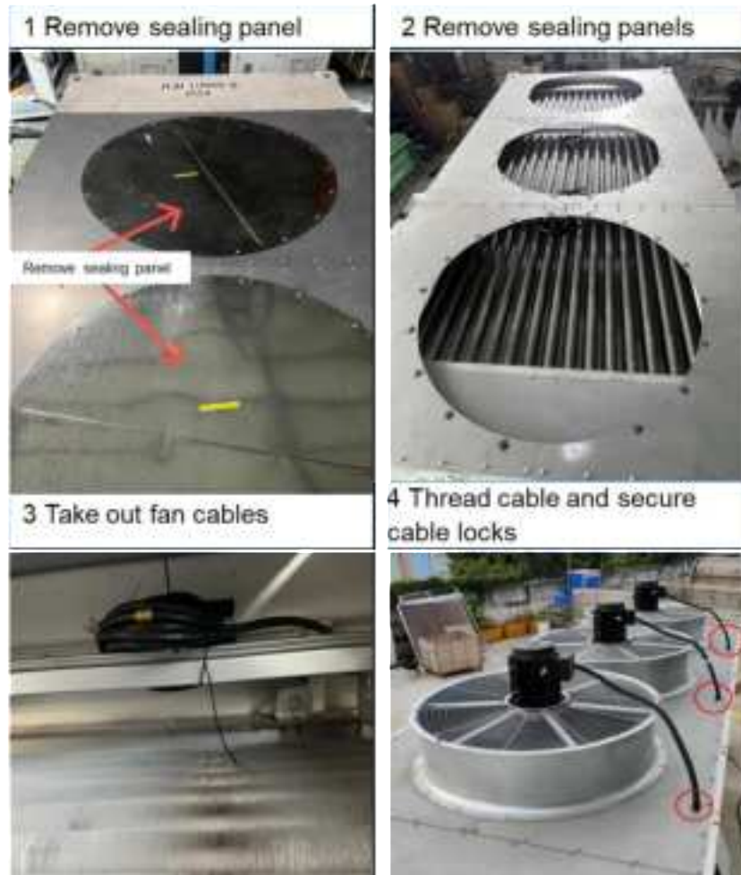
Figure 7-5 Schematic for Removing Fan Sealing Panels
