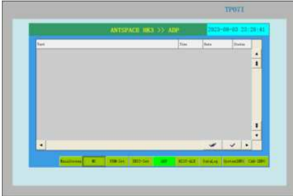
Figure 7-30 Alarm display interface
