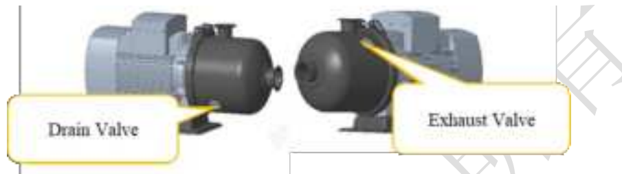
Figure 7.9 Recharge Pump Drain and Bleed Valve
